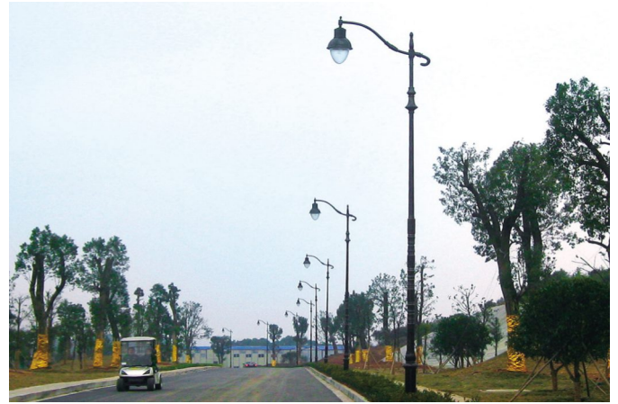
Hunan Changde Ecological Park Road Project
